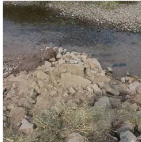
An installed rock groyne.
