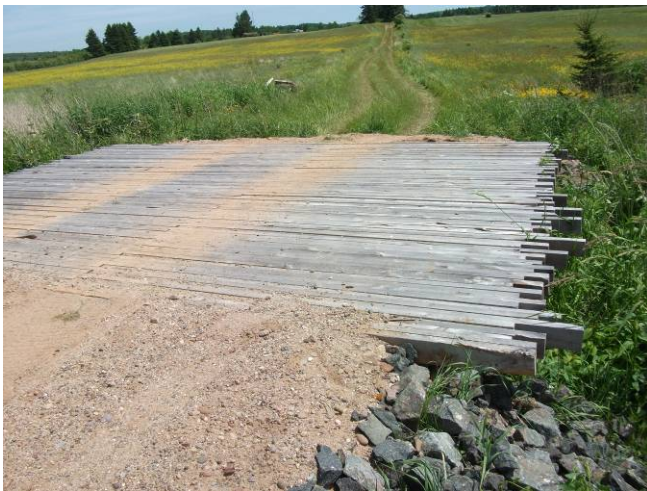
Photo 2: Picture of the bridge built at Kurihipi Station.
