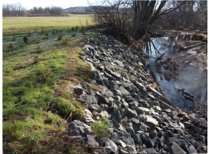
Picture 3: The smaller bank stabilized by the KWRC in 2009.
